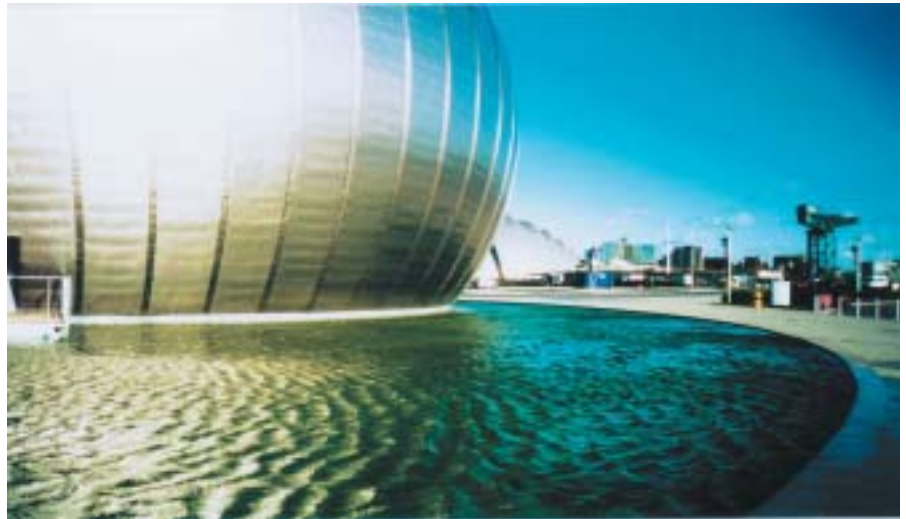
Example waterproof lining at Science park, Glasgow
